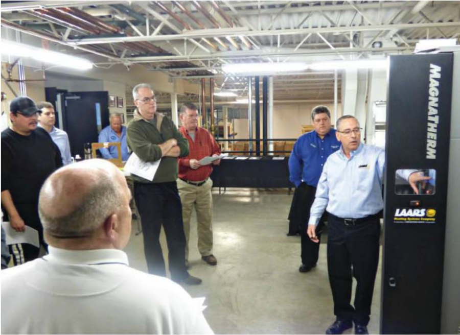
Laars National Training Manager Steven Moruzzi (far right) conducts a session on a working MagnaTherm boiler at Michel Sales' headquarters. The manufacturers rep has increased its training capabilities in concert with its investments in commercial products.
